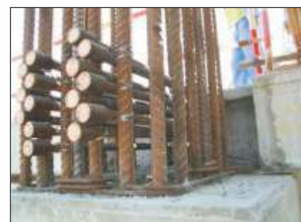
Beam to column connection
