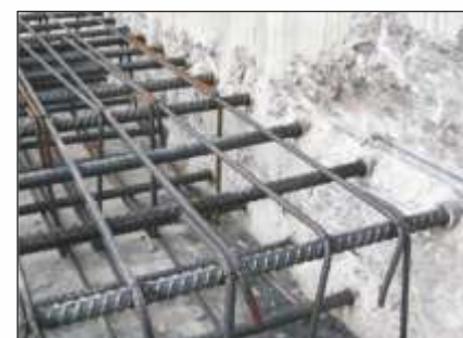
Wall to slab connection
